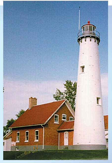
Tawas Point Light (State Historic Preservation Office)
